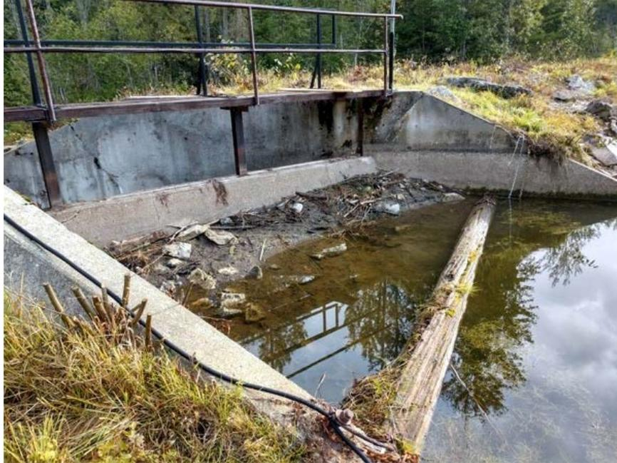
The spillway for the Cambridge Creek Reservoir Dam has been found to be under-sized for significant storm events, which may cause failure of the dam.
