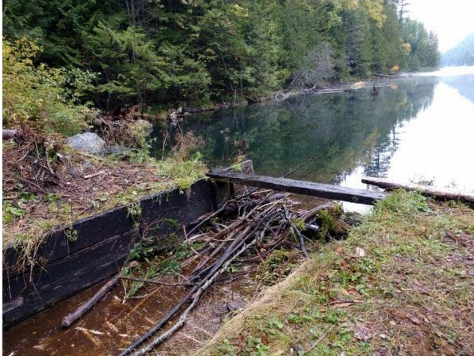
Beaver regularly block the poor-quality wooden spillway for the Violin Lake Dam. Water is leaking under the spillway, which may cause the dam to fail.
